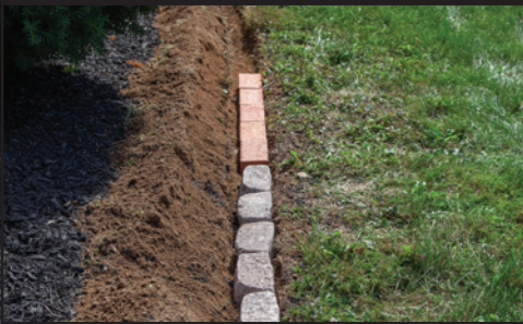
T5 - Trenching 5" x 5"
